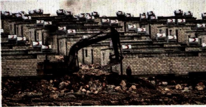
The construction of briquette houses continues in Idlib, Syria, Jan. 28, 2021.
