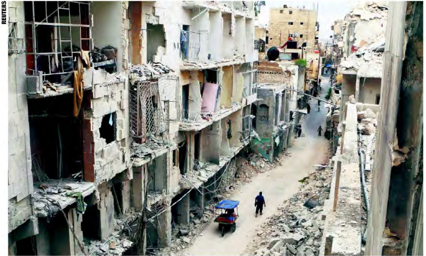
Desperate residents walk among the damaged buildings in the Old City of Aleppo, Syria, May 5.
